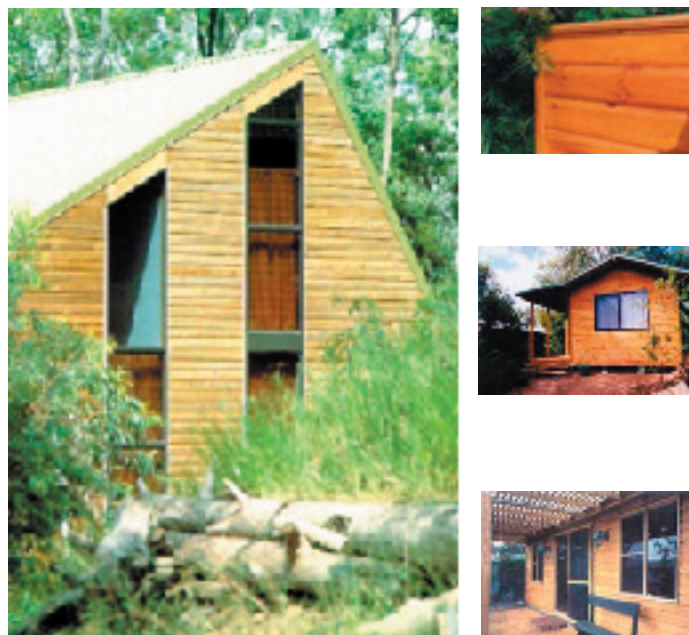
Timber clad homes made with CCA-treated products.
