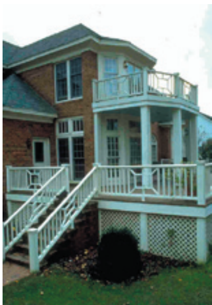
LOSP-treated external joinery, benefiting from a well-maintained paint coating
