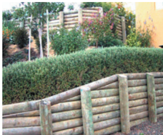
Sound treated timber retaining walls
